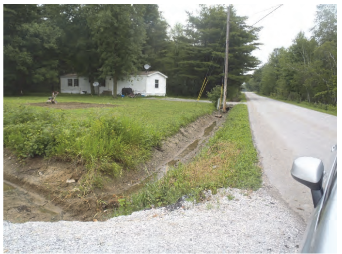
Photo 2. More raw ditch, agricultural drainage ties directly into roadside ditch at lower left corner of photo
