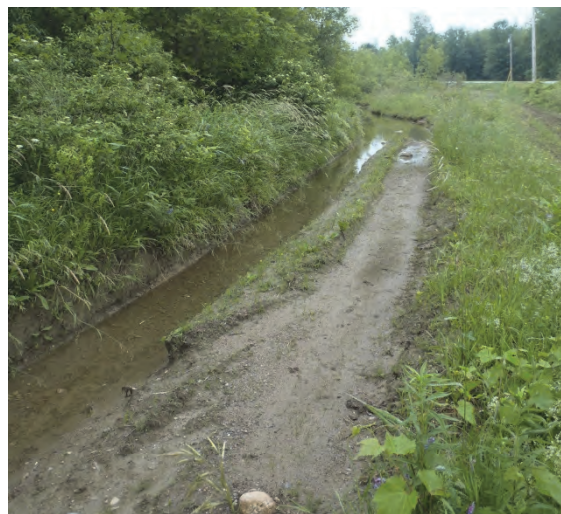
Photo 1. Flooded private access road; note 1' high bank on left side which seems to show some signs of erosion
