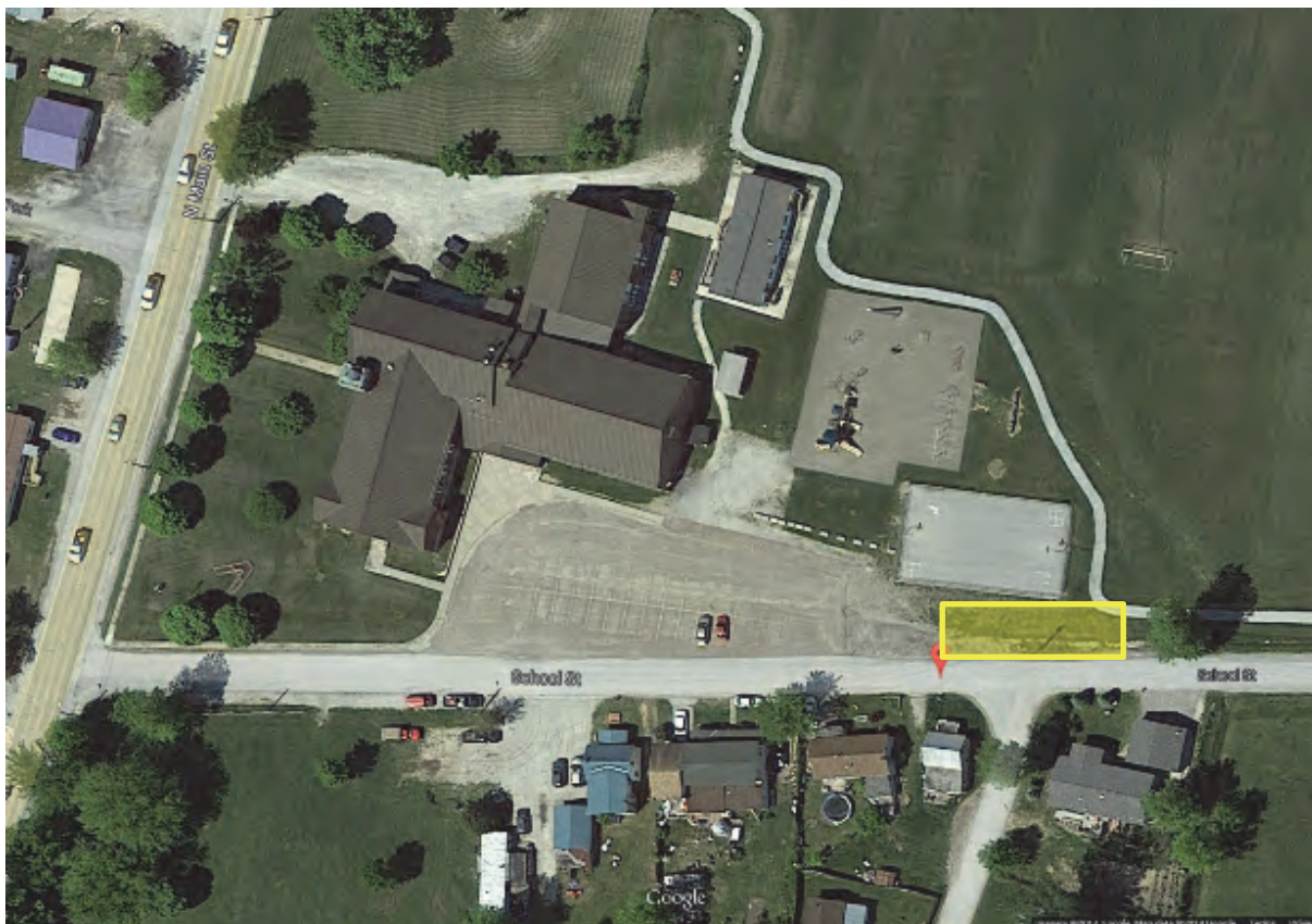
Figure 4. Aerial view of Alburgh School site which has a significant amount of unmanaged impervious cover, including the building roof and parking area. A potentially suitable area for a stormwater management practice is highlighted in yellow.
