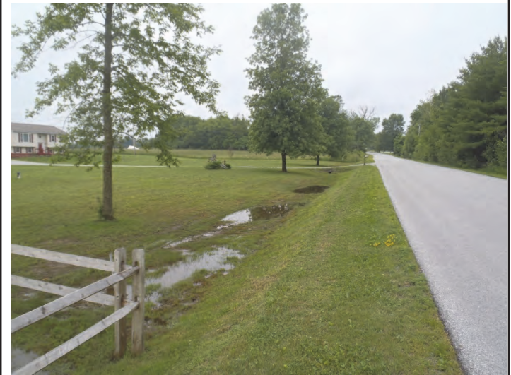
Photo 2. Poor drainage along the eastside of Greenwood Rd
